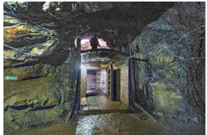
At Wlodarz very little of the complex has been concrete-lined. Here, just the entrance to a side chamber has had the treatment. Photo Chris Rayner
